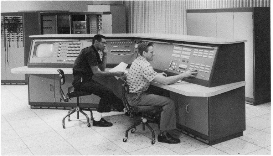
SDC technicians operating special-purpose communication systems built by SDC for the SSRL: the RL-101 (left half), providing real-time communication between the Philco 2000 and many simultaneous experiments; and the RL-102 (right half), enabling participants in an experiment to intercommunicate and observers to hear and record subjects' responses.
