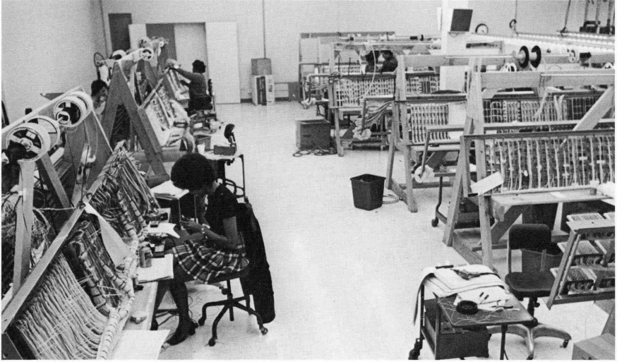
SDC built its first hardware laboratories in the early 1970s for the Los Angeles Sheriff's Communication System. ( Above ) Assemblers build wiring harnesses for the switching subsystem. Production line of communication consoles is seen below.
