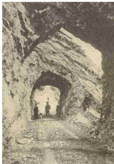
Photograph by Clinedinst. Shoshone Project. Wyoming Park wagon road, showing wonderful tunnelling work on the new wagon road from Cody, Wyo., to the National Park via the Shoshone Dam.
