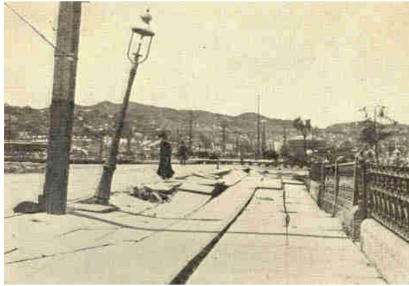
Earthquake at San Francisco, April 18, 1906. Upheaval of sidewalk at Eighteenth and Capp Streets.
